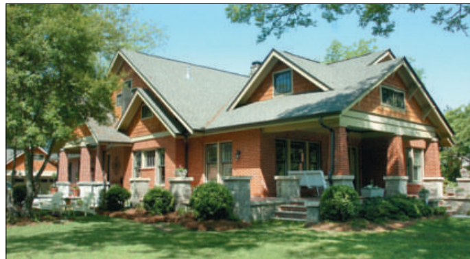
By raising the roof line 18 inches and adding to the back of the house, this bungalow grew to a five-bedroom, 5½-bath home.
